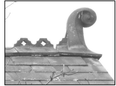
Detail of decorative terracotta finial to the station roof, 2006. A common design element on the wooden built 'Derbyshire Lines' stations. (Philip Cousins)
