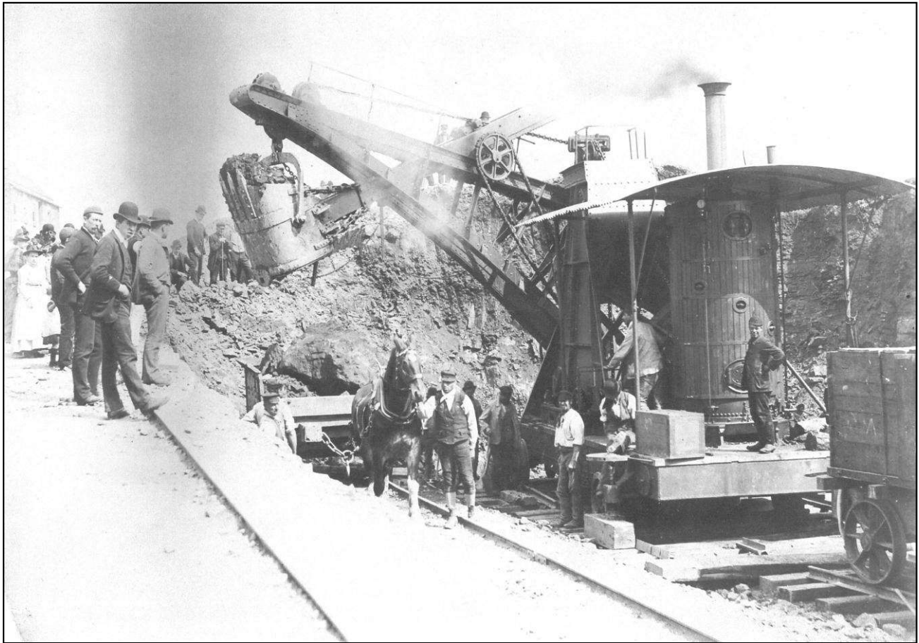
A 'steam navy' at Nags Head cutting, Staveley, 1890. Though not a Brimington scene we could not resist printing this photograph of a steam navy at work creating the cutting, now in-filled, in the vicinity of the Nags Head public house, Staveley. Steam navvies were occasionally called 'steam devils' in contemporary newspaper reports. The photograph was taken by a Mr. Bowmer, who was a general dealer and photographer, with a shop on Staveley's High Street. Here the photograph was displayed in his shop window for many years. Note the spectators and the lack of any fencing on the works. The road into Staveley was carried over the cutting by an iron bridge in the vicinity of the Nags Head. On closure of the line the bridge was underpinned and filled in, along with the cutting. The iron sides of the bridge were burnt off. About 25mm can, however, still be seen protruding at the edge of the footway, opposite the public house. (Courtesy Fred Wood)
